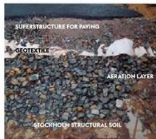
Layers of a planting bed with Stockholm structural soil.
